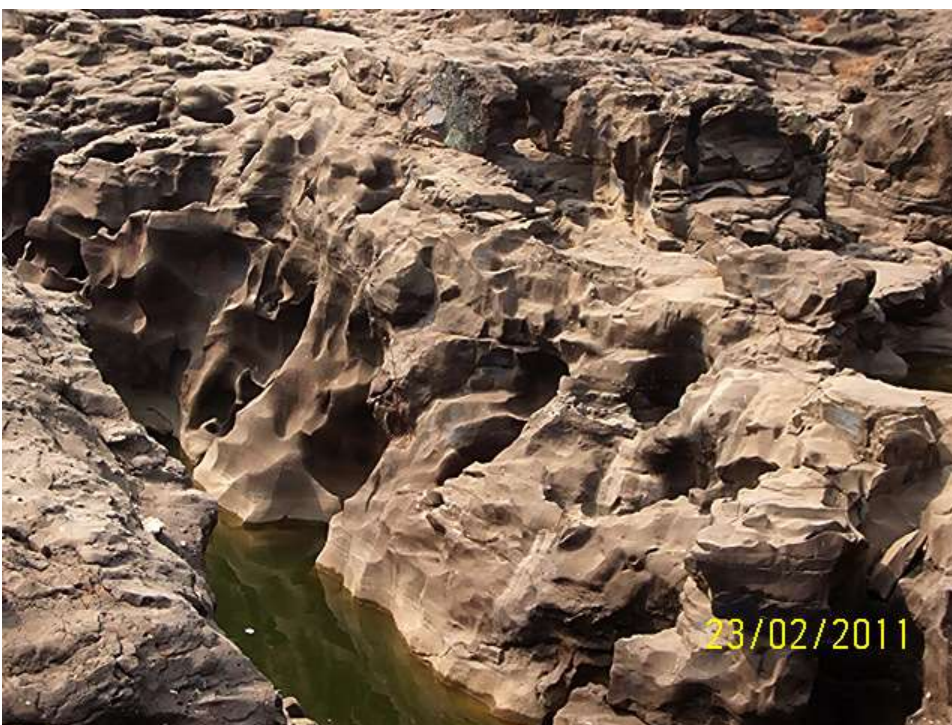
Erosion of river Kukdi, Nighos
